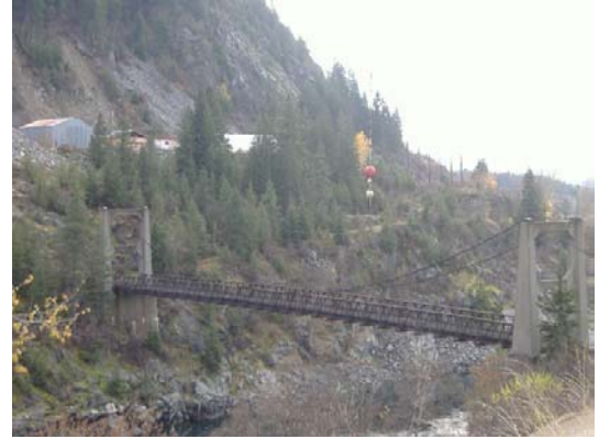
Fig. 12. The Brilliant Suspension Bridge.
